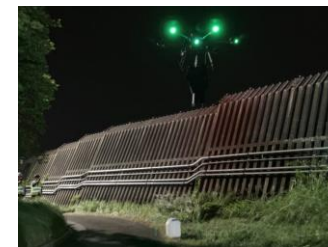
High-altitude inspection using drones
