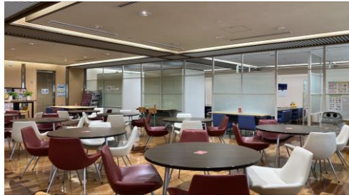
Conversion to LED lighting
